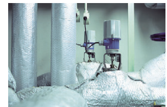
Air conditioning system
