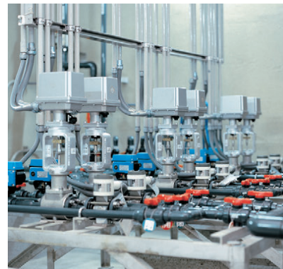
PSN installed in a water treatment plant
